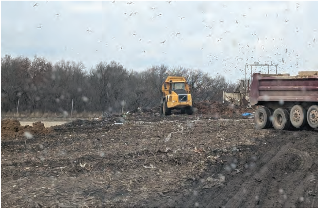
Wood waste making for good travelway over ADC
