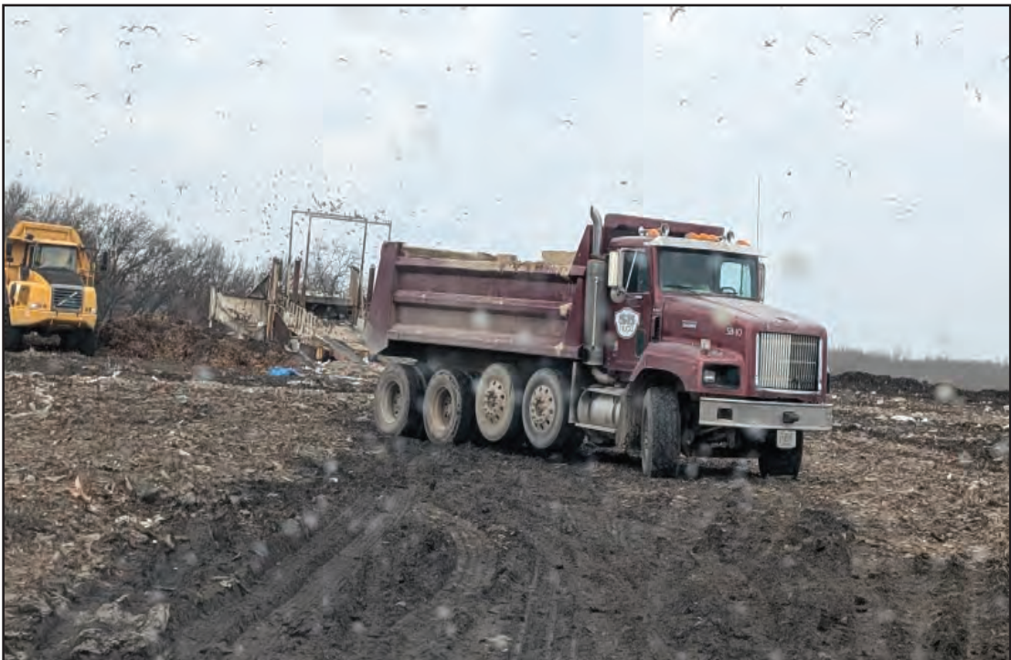
Travelway rough and mucky where wood waste has been lost
